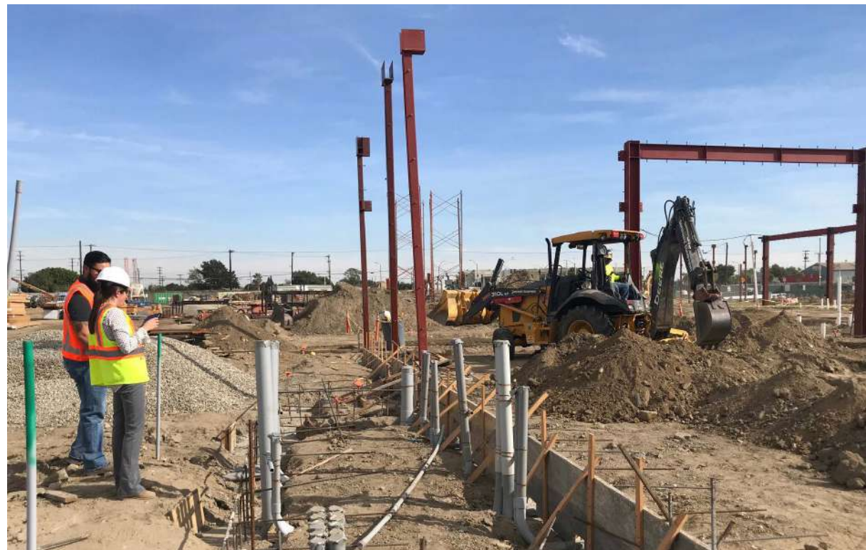
Freedom Plaza Construction
