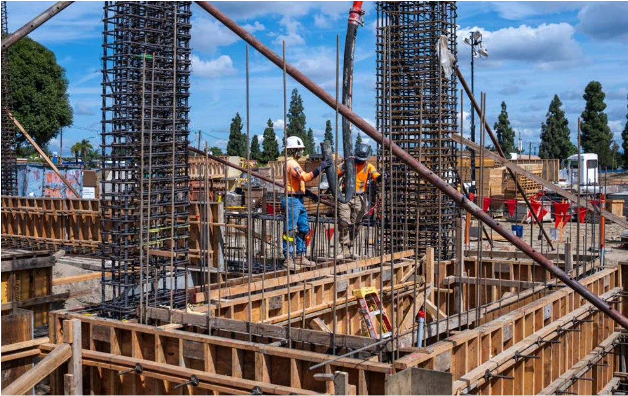
The Walk Construction
